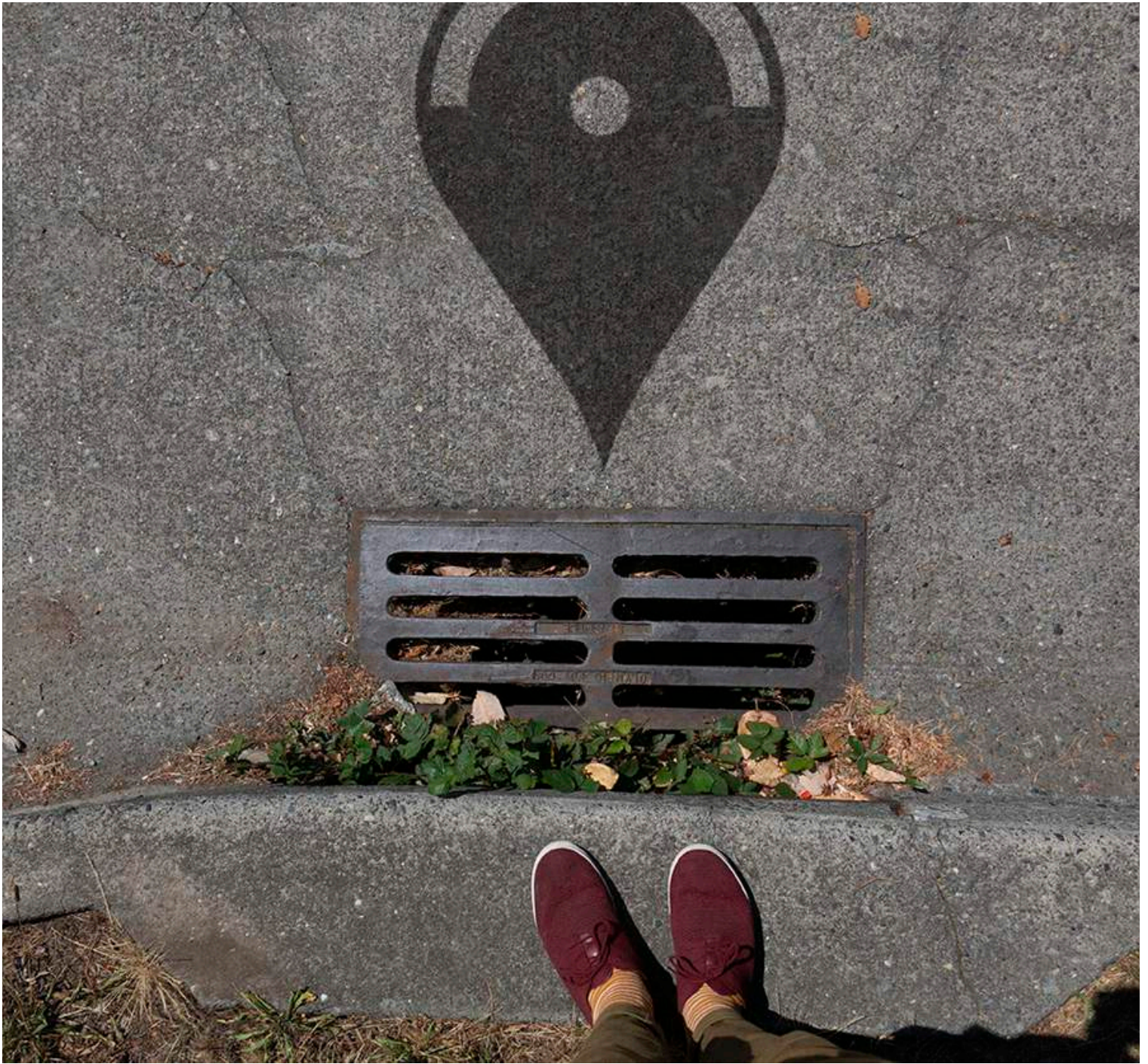
This is a representation of a potential drain activation using hydrophonic coating paint (water activated paint).
